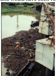
breached. The span between each steel pier was not long enough to allow the debris to pass the bridge without "clogging" the span.
